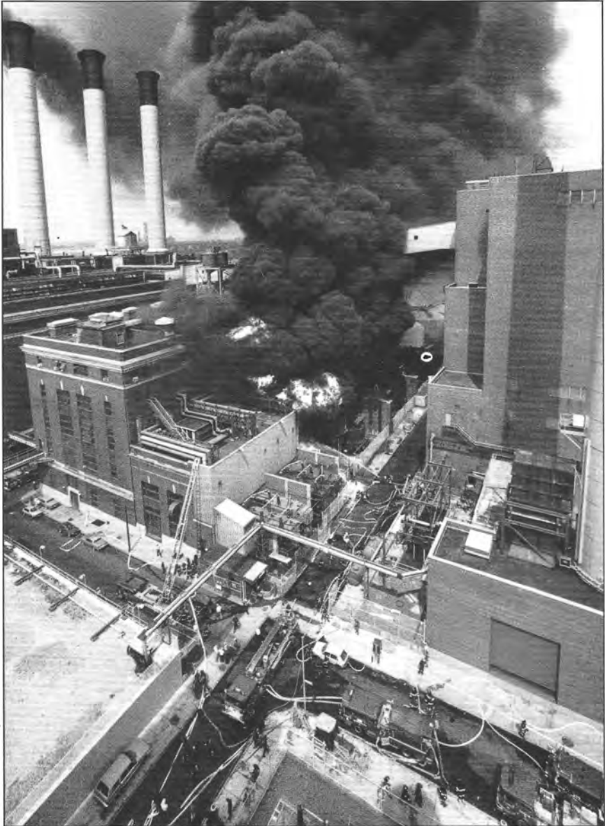
An explosion of unknown origin started this fire on June 14, 1988, in the transformers of a Con Edison Electrical generating plant in Brooklyn. Members of Haz-Mat took air samples to determine if PCB's or other toxins were emitted.
