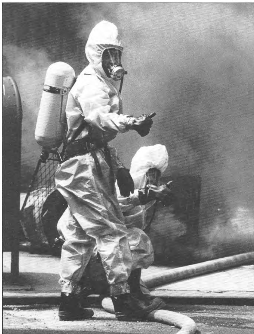
Two members of the Haz-Mat unit in protective clothing signal their readiness before descending into a manhole to fight a transformer fire at Park Avenue and 78th Street in Manhattan. Photo: Vic DeLucia/The New York Times
