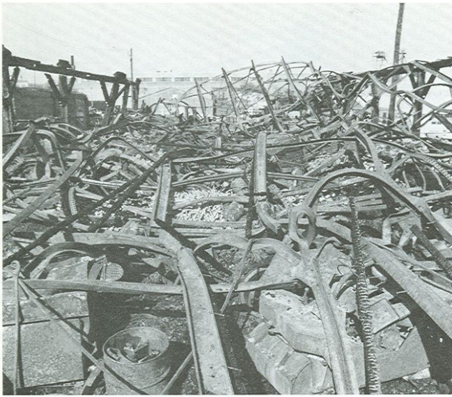
A jumbled mass of twisted steel and debris are all that remain of the large warehouse. Members of L.155 and E.315 were repositioned shortly before the collapse, averting possible serious injury.
