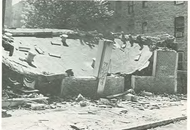
The roof section of the laundromat which sustained a dangerous unsupported (one portion hanging free) lean-to type of collapse. Photo by A. Guerriera, F.D.N.Y. Photo Unit
