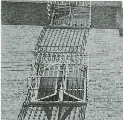
In Williamsburg, Brooklyn, fully barred windows have been installed as high as the fourth floor in some buildings. Bars come in a variety of styles: in photo above, left, note encased air-conditioner; center photo shows installation designed to allow windows to open out. Building in photo at right is particularly dangerous because the random installation of the bars means that each apartment is different.
