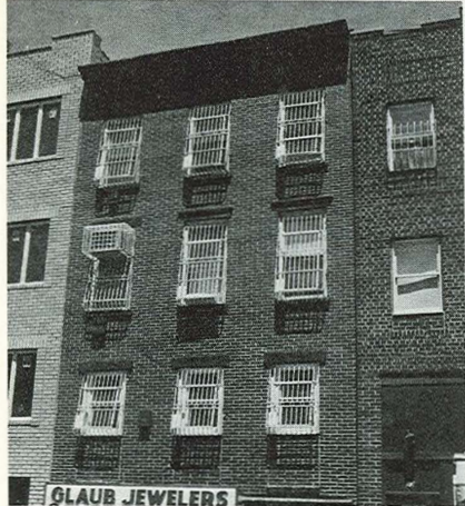
In Williamsburg, Brooklyn, fully barred windows have been installed as high as the fourth floor in some buildings. Bars come in a variety of styles: in photo above, left, note encased air-conditioner; center photo shows installation designed to allow windows to open out. Building in photo at right is particularly dangerous because the random installation of the bars means that each apartment is different.
