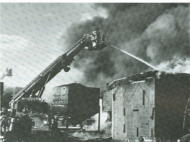
Through doors and other building interconnections, the fire quickly traveled through the rear extensions at the exposure 2 end of the complex. There, too, a tower ladder had a large-caliber stream in place. Photo by Jim Regan
