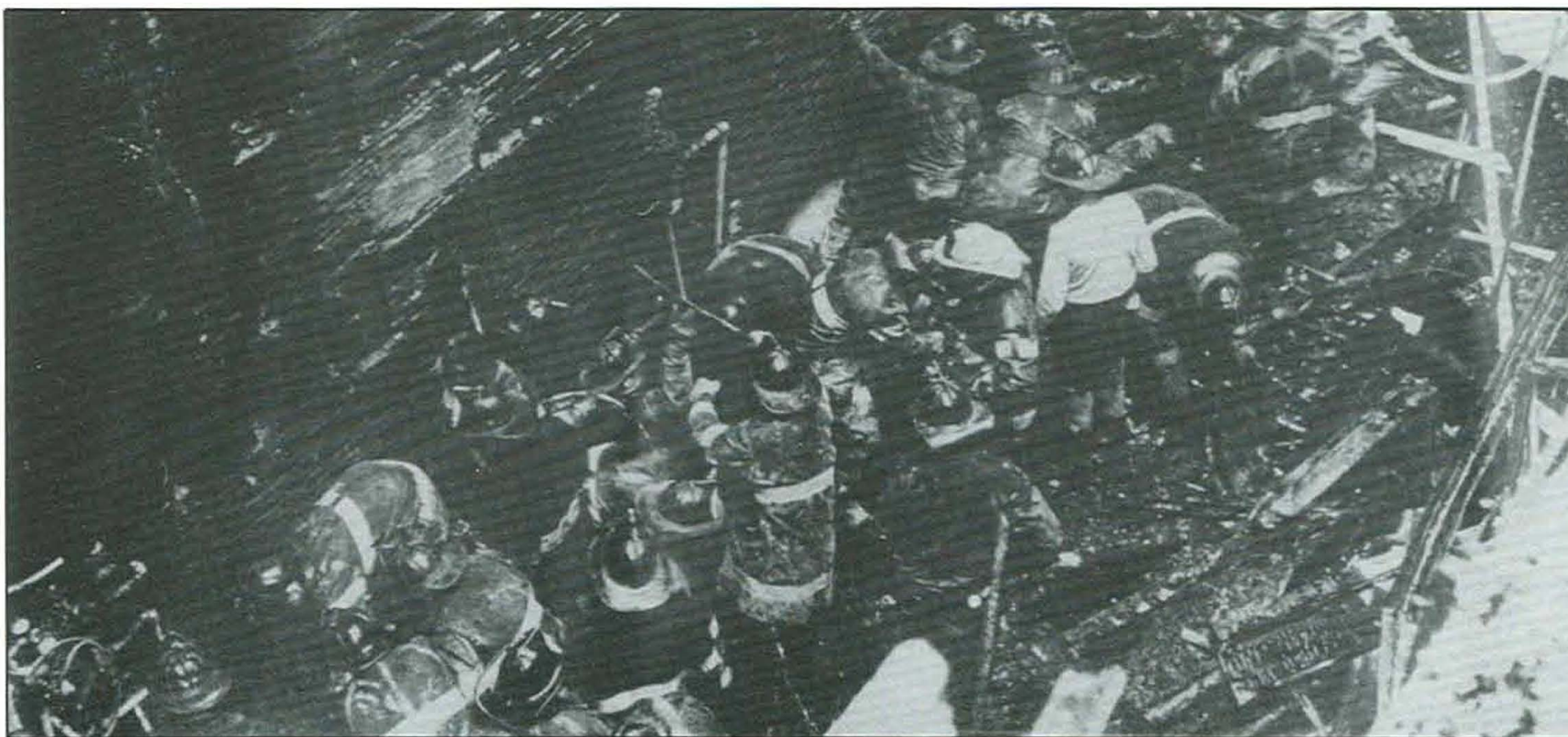
Masonry floor collapse caused the death of 12 firefighters and officers at the 23rd Street fire.
