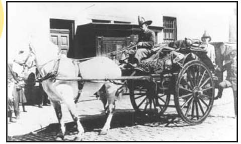
Engine 18 posed with an early version of the “modified” hose tender. Originally, only the driver rode on the hose tender. Seats were added over the hose reel and a small step was added to provide riding positions for engine company personnel.
