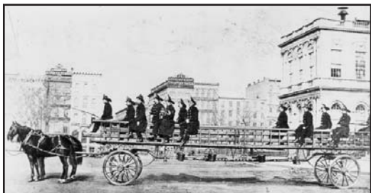
The earliest apparatus used by the Department had minimal riding positions. Although Ladder 1's entire on-duty crew of 12 posed on their apparatus in front of City Hall for this photo, only the driver and tillerman actually rode on the apparatus to fires. There are no other riding positions or running boards on this apparatus. The remaining members ran alongside the apparatus, the origin of the term “run,” when referring to a response.
