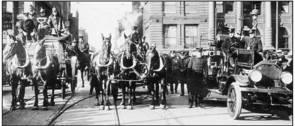
As the size of both motors and pumps was reduced, it became possible to add a hose bed to pumpers. Engine 205, shown here at a symbolic "last horse-drawn run" is replacing both its horse-drawn steamer and hose wagon with a single motorized pumper. Engine 205 was the last unit to be regularly assigned horse-drawn apparatus, which were replaced in 1922 by an American LaFrance pumper.
