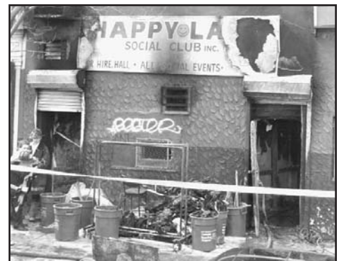
The actual firefighting operation at Happy Land required the services of only a first-alarm assignment to control. The subsequent overhaul, investigation and removal of victims led to the assignment of 50 units.
