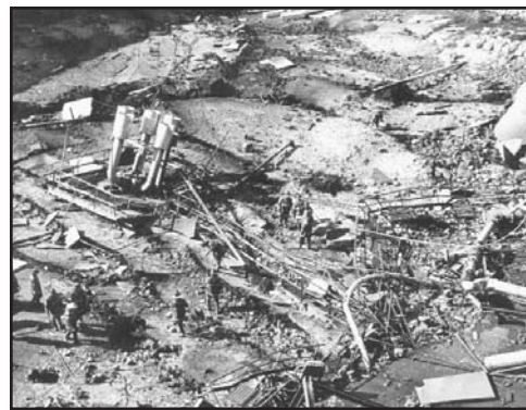
The concrete roof of the Staten Island gas tank collapsed, killing and burying the workers inside.
