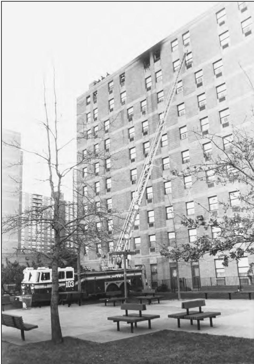
Tragic fires, such as the one at Vandalia Avenue in Brooklyn, brought about sprinkler law reform through Local Law 10.
