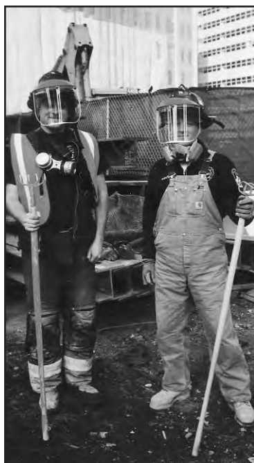
(Above) Full-face shield protection-- Firefighters sifted through debris containing ammunition.
