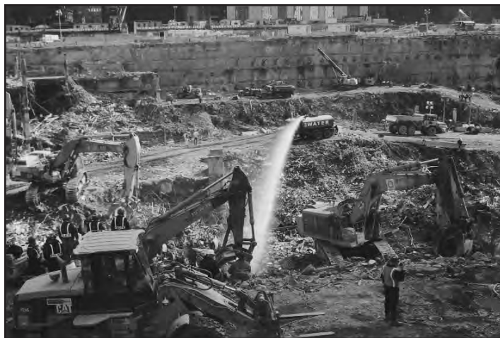
(Above) Dust suppression--Water tanker sprayed hot spot in debris field.
