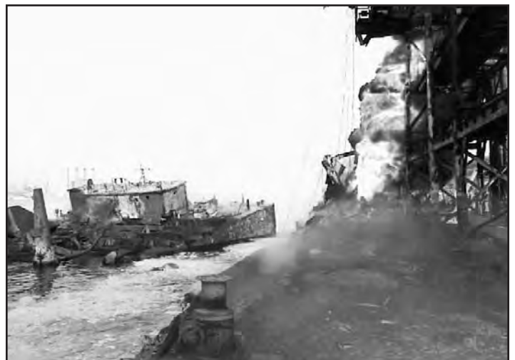
Remains of the shattered gasoline barge lie in the background as flames pour from the ruptured product manifold.
