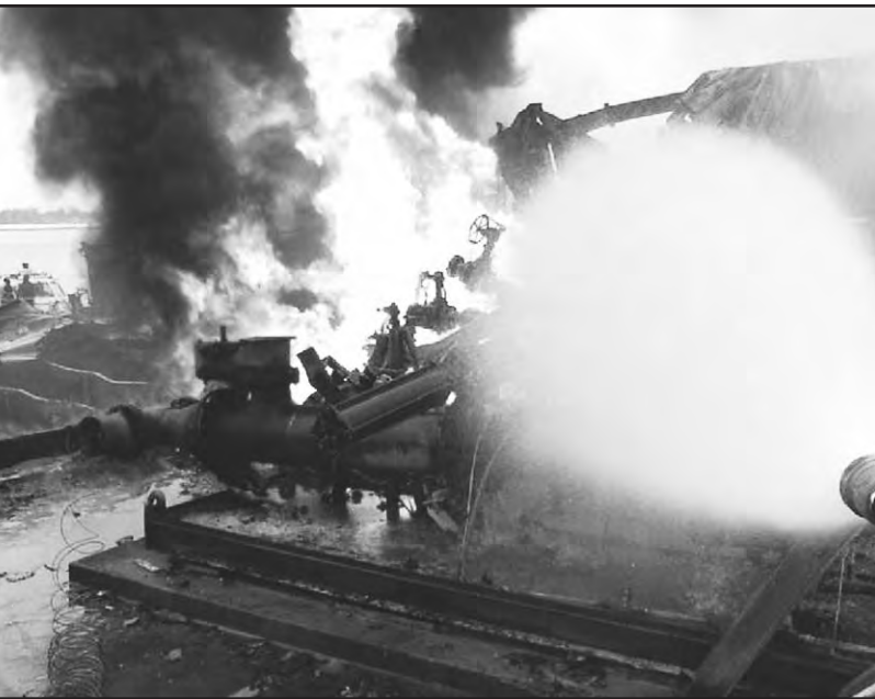
One of the hand-lines that was lashed in place provides cooling water on pipe manifold to prevent further damage to product lines.
