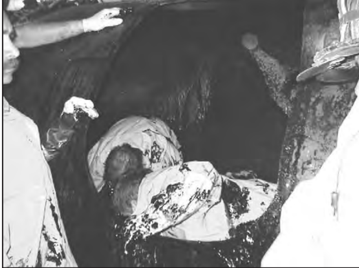
FFs John O'Connell (left) and Michael Davis of Rescue Company 3 prepare to remove the first of the overcome workers after entering the tank through an opening that had been created with a sawzall. Note use of disposable PVC Level D suits instead of bunker gear. The heavy #4 oil necessitated that any contaminated clothing be disposed. Flash point of this oil is 125 degrees.
