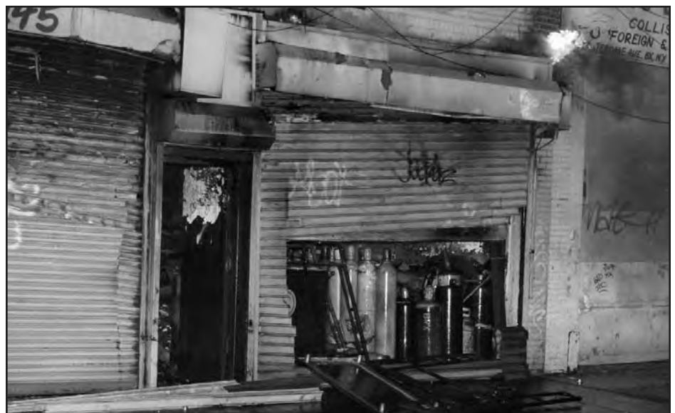
These cylinders (containing oxygen, acetylene and argon) were found by FDNY members. Note the fire coming through the parapet, near the top of the roll-down gate.
