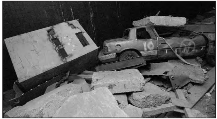
The debris pile, which ran from tunnel wall to tunnel wall, featured numerous scattered vehicles, including a leaking tanker-truck.
