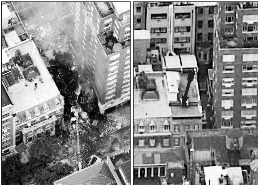
(Left) Water is poured on remains of four-story collapsed building. The incident went to six alarms before being brought under control. A buried victim was brought out alive, but he died later in the hospital. (Right) Dr. Nicholas Bartha's brownstone (arrow) before the gas explosion and fire reduced it to rubble.
