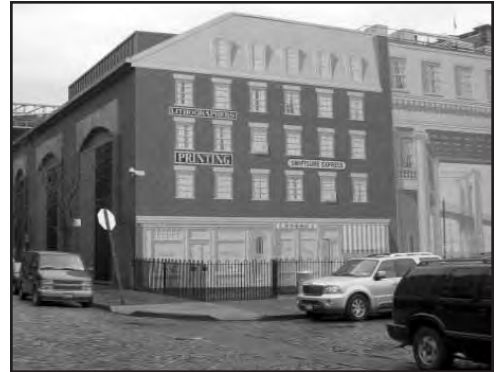
Photo #1--From the exterior, the Con Edison substation appears to be a five-story building.
