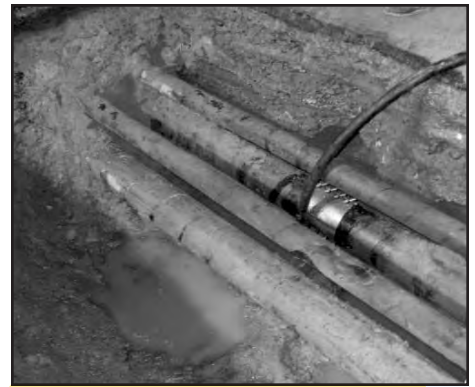
Photo #7--Exposed underground feeder lines.
