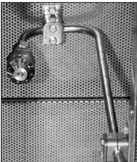
Unique water mist nozzle with multiple orifices and stainless steel piping.
