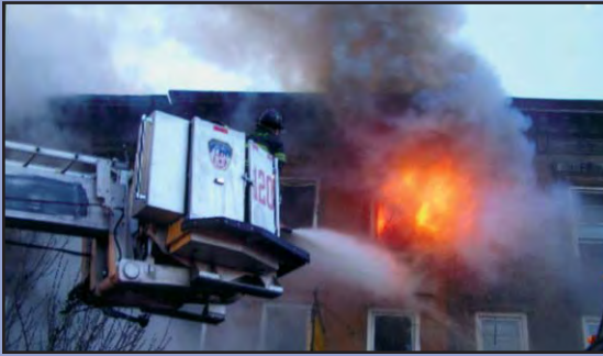
Brooklyn Box 33-845, 2148 Fulton Street/Rockaway Boulevard, January 4, 2008. Ladders 120, 111 and 103 were among the units operating at the incident.
