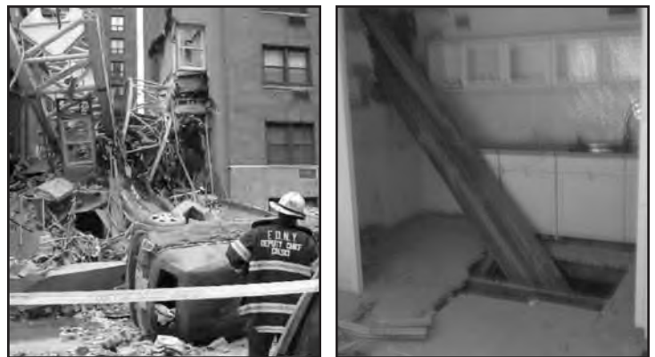
Photos #6 and #7--In photo on left, Chief Cresci examines the damage (which included a major water leak in a basement) within the 50th Street Sector. The photo on the right shows the 30-foot I-beam that pierced the roof of 306 East 50th Street.
