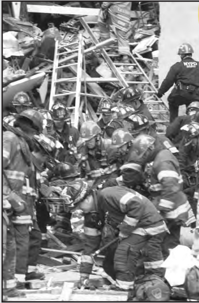
FDNY member--hit by roof sheathing--is removed from the crane collapse site.
