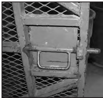
Photo #16--Landing gate lock.
