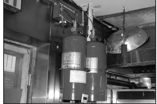
(Left) Portable (Class K) wet chemical fire extinguisher with unique wand applicator. (Above) Wall-mounted releasing mechanism and pressurized wet chemical cylinders. (Right) Class K (wet chemical agent) portable fire extinguisher pictogram.
