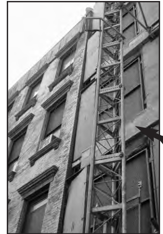
Photo #26--The floor number (arrow) is spray-painted on the building.
