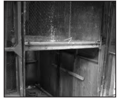
Photo #18--Open landing gate.
