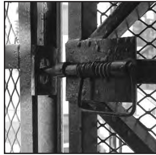
Photo #17--Spring-loaded latch.
