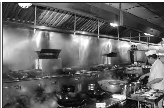
Commercial wet chemical fire extinguishing system.
