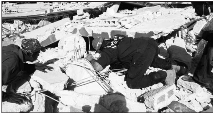
Photo #5--A Hasty Search is one that is fast-paced and methodical. Members work in an assigned area where it is believed that trapped civilians can be successfully rescued from an entombed structure.
