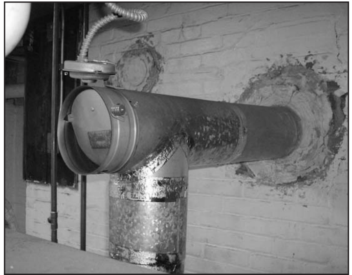
A draft inducer can be placed in-line or used as an elbow. In this installation, the draft inducer is placed at a right angle to the chimney.
