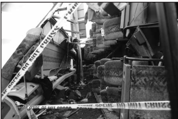
Photo #2--Due to the impact of the accident, overhead luggage racks and bus seats became separated from the bus.
