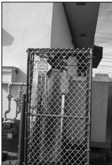
(Far left) Photo #4--Interior installation. The arrow is pointing to CO2 supply line going to the exterior of the building. (Left) Photo #5--Typical exterior installation of Dewar-type CO2 cylinder. (Above) Photo #6--Top of cylinder. Note ID plate attached to the top of the cylinder. The arrow is pointing to the total contents in lbs. when full (387 for this size).
