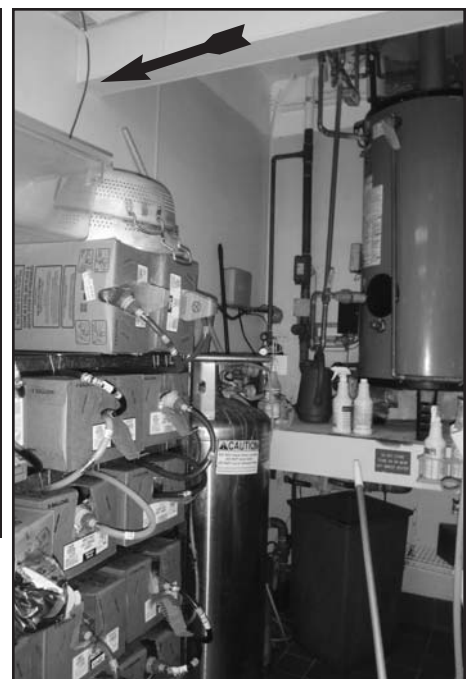
(Left) Photo #1—Typical size Dewar-type cylinder, capable of holding 387 lbs. of liquid CO 2 . (Above) Photo #2—Top of cylinder. Note the numerous shut-off valves. The arrow is pointing to the gauge in the center, which shows how much CO 2 is in the cylinder. (Right) Photo #3—Interior installation. The arrow is pointing to CO 2 tubing going up to the ceiling.
