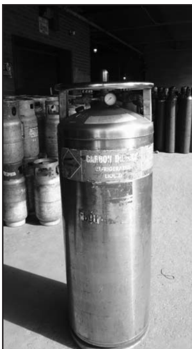
(Left) Photo #1—Typical size Dewar-type cylinder, capable of holding 387 lbs. of liquid CO 2 . (Above) Photo #2—Top of cylinder. Note the numerous shut-off valves. The arrow is pointing to the gauge in the center, which shows how much CO 2 is in the cylinder. (Right) Photo #3—Interior installation. The arrow is pointing to CO 2 tubing going up to the ceiling.
