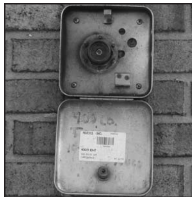
Photos #7 and #8--Exterior fill connection shown in the open and closed positions. Often the cylinder will be located opposite this wall as long as there is access to this location for the supply truck. This would be a clear indication that CO2 cylinders are located inside.
