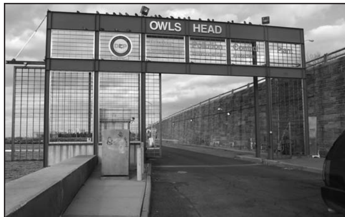
Entrance to Owls Head (DEP) Water Pollution Control Plant in Brooklyn.
