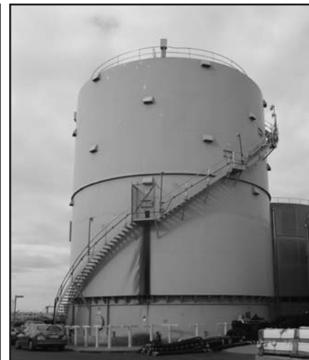
(Left) Mechanical screens are an entanglement, as well as a confined space, hazard for facility personnel and FDNY members. They are used in primary wastewater treatment processes. (Center) Aerobic wastewater treatment tanks are used as a secondary process. (Right) Biogas storage poses flammability and toxicity hazards.
