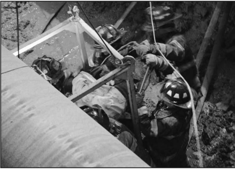
FDNY members positioning and securing the freed sandhog into the man basket for removal from the excavation.
