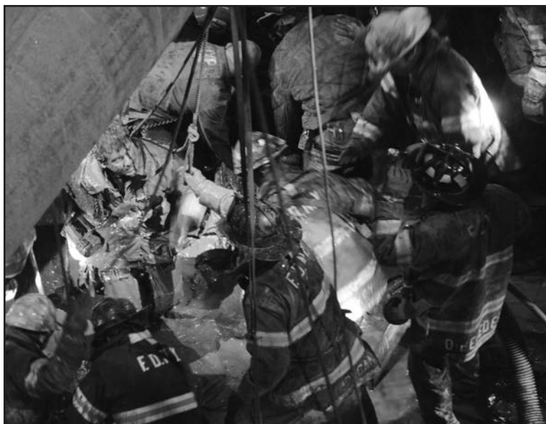
Trapped sandhog up to his chest in Bull's liver (shown slightly below and to the left of center) secured to rope and harness assembly. Firefighters worked tirelessly for more than four hours trying to free him. photo by CTU
