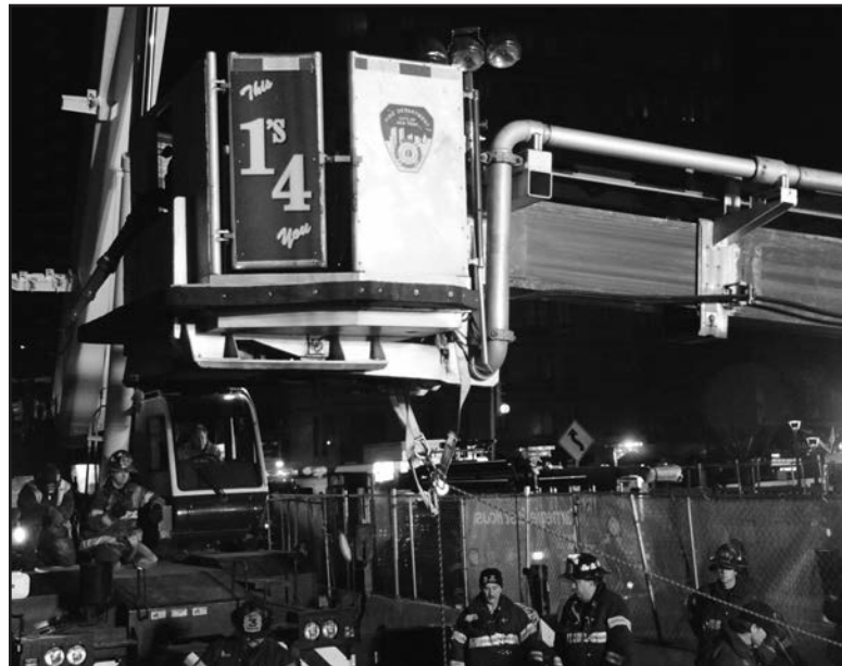
Tower Ladder 14's bucket was positioned over the large street opening and used as a high point. Also note the crane operator and crane that had a man basket attached to it, located just south of the bucket.
