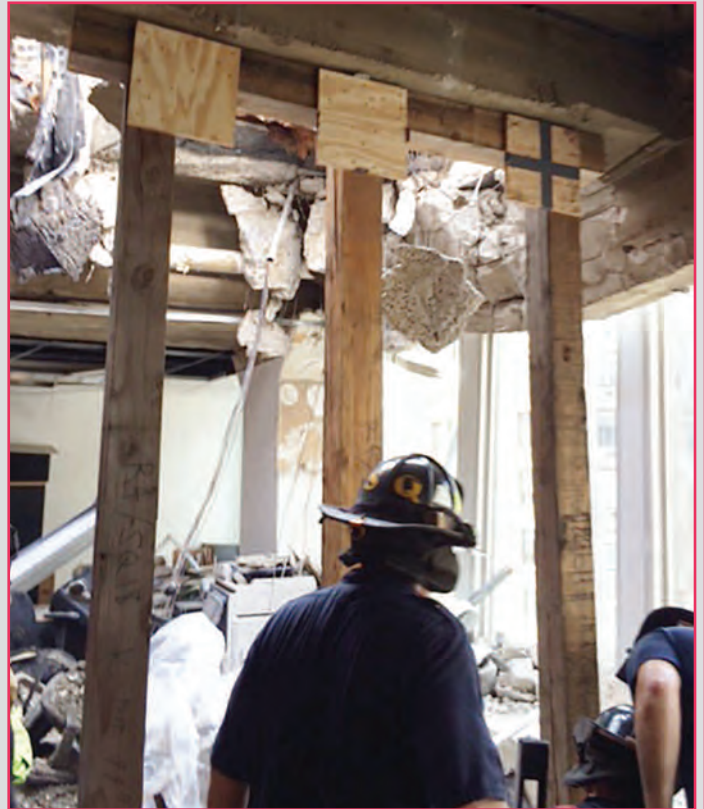
Members working on 15th floor, installing a three-post vertical shore.
