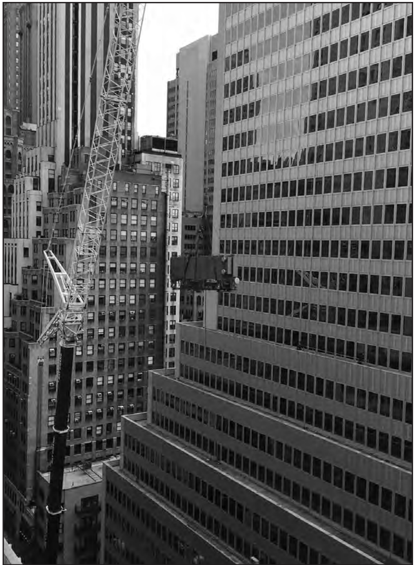
Crane operator was hoisting the chiller to one of the top three floors to the mechanical equipment room at 261 Madison Avenue. Approximately halfway up, something went terribly wrong. See photo on facing page.
