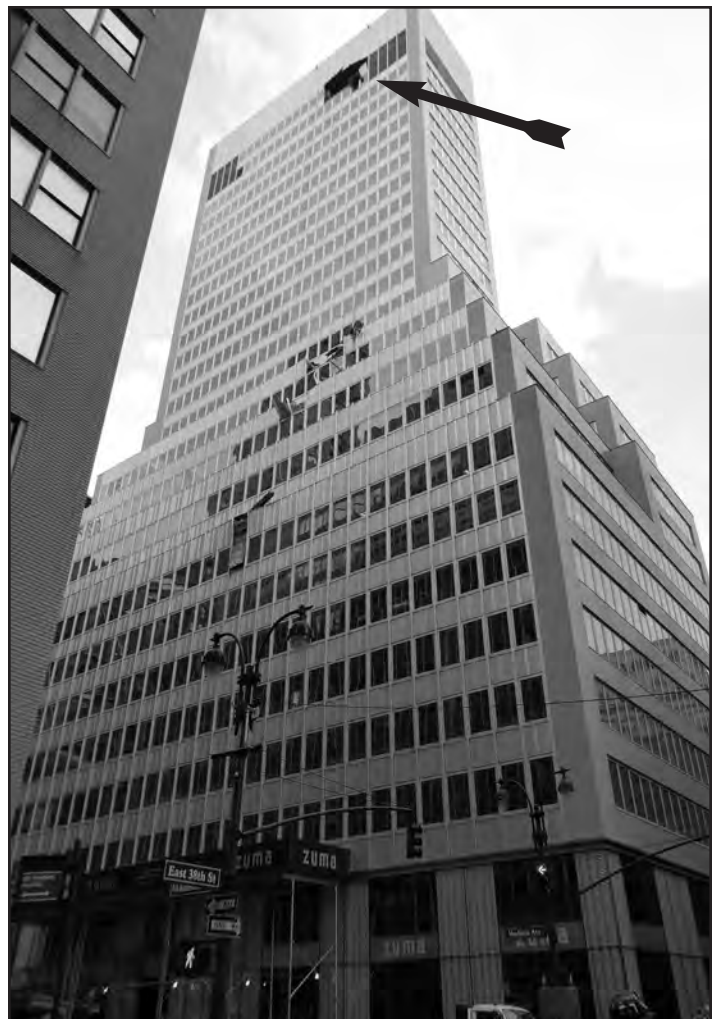
Damage to roof setbacks and facade is evident in this photo. Arrow denotes mechanical equipment room entry point for the water chiller.
