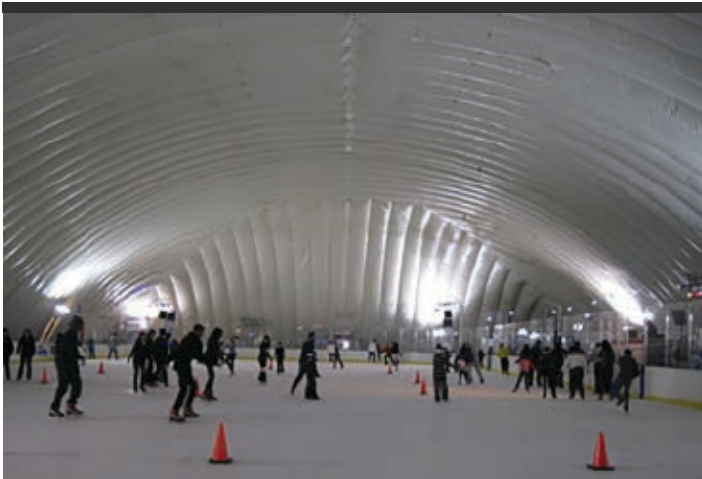
Photo #2—The interior of the City Ice Pavilion, which is built on a roof-top. Note the high glass along the boards, which could cause damage to the fabric during high winds if not maintained properly. It will be difficult for people wearing ice skates to evacuate.
