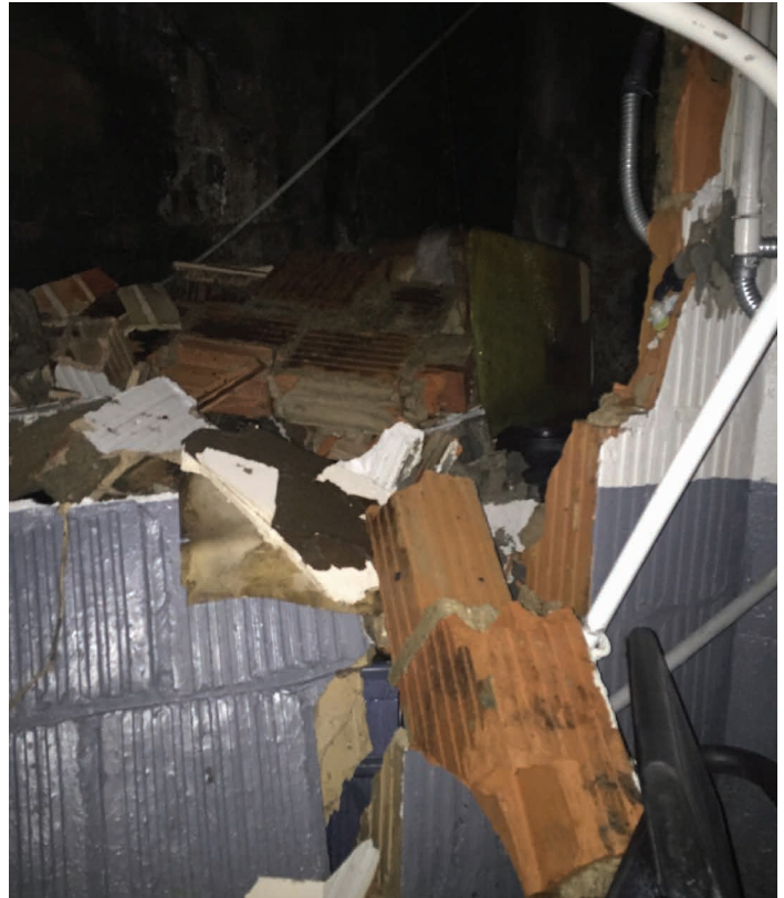
Basement walls blown down by the force of the explosion. Except where noted, all photos by Deputy Chief Joseph N. Carlsen, Division 3 Commander.
