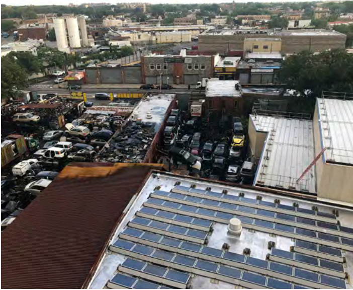
The burning junkyard cars threatened nearby commercial buildings.
