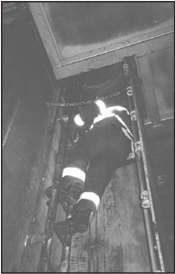
Man-way ladder, adjacent to car/truck elevator.
