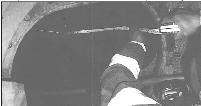
Baffle plate (measuring 12 inches high) inside confined space. Note: All photos were taken during critique operations, after the incident and after the ship was made safe.
