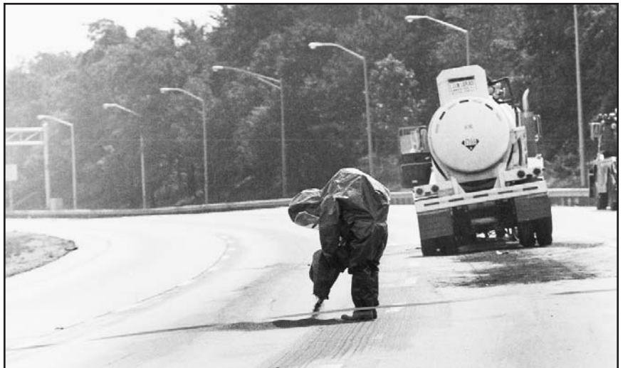
Rescue 5 member spreads Speedi-Dri to help absorb some of the remaining spill.
