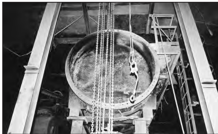
(Above) Prior to the the fire in the basement involving titanium rods and a subsequent electrical explosion at One New York Plaza on December 1, 2001, several fires had occurred within this large-diameter "chiller" unit. A subcontractor was in the process of dismantling the unit.
