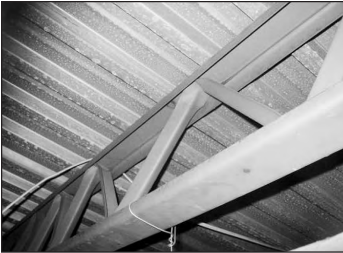
Photo #2--Trusses may be constructed with bars or, as shown here, cold-formed steel sheets.
