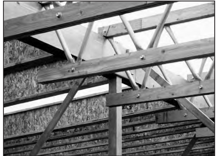
Photo #3--Another type of lightweight truss consists of wooden chords and tubular steel webs.
