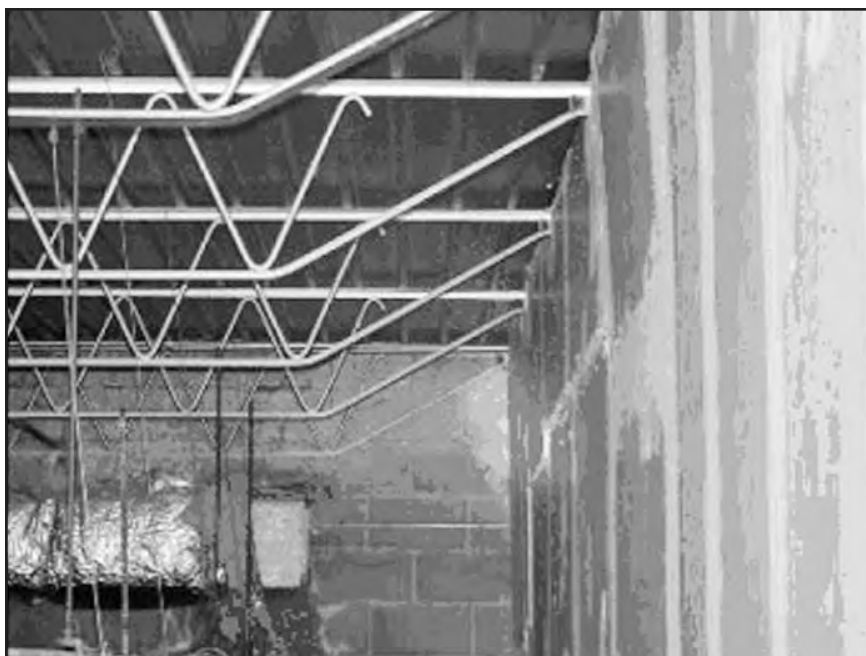
Photo #1--Typical bar joist construction.
