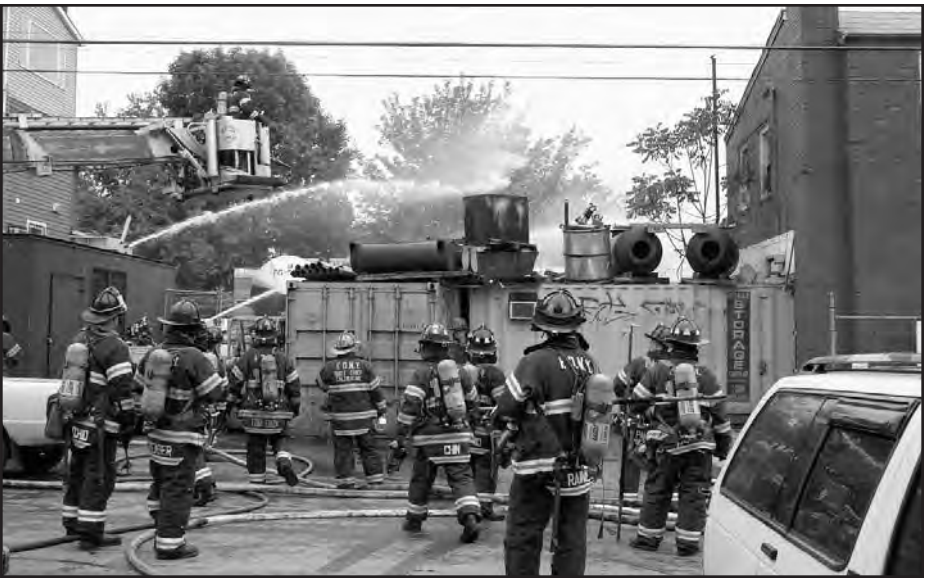
The two tanks in the storage yard had exploded, which caused substantial structural damage and a partial collapse on the exposure #2 side of the fire building, as well as the roof of the 25- by 75-foot extension at the rear.
