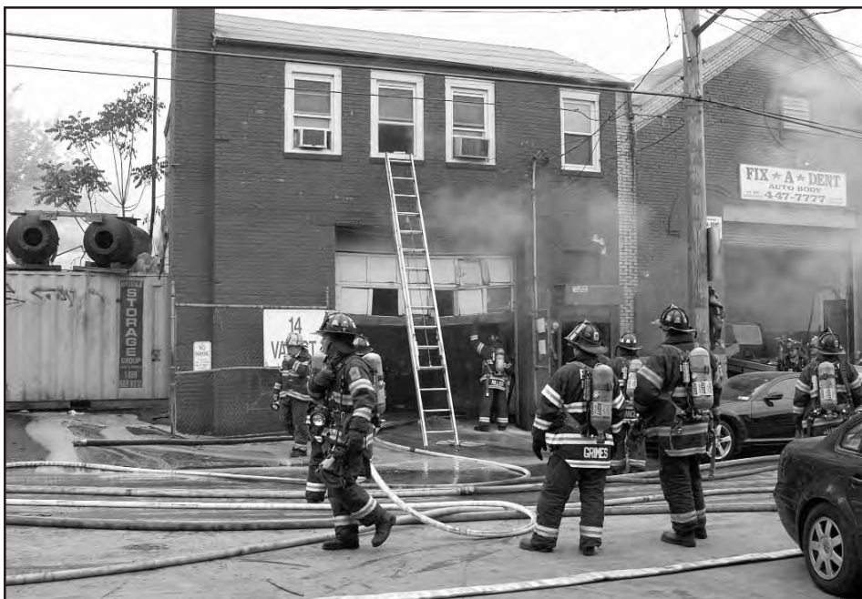
Site of Staten Island Box 22-0399, 14 Van Street. This irregular, two-story, 20- by 60-foot, brick-and-joist structure featured a one-story brick extension at the rear. Exposure #4 is an attached, two-story, peaked-roof brick structure used as an auto repair shop. Exposure #2 included two large, horizontal exterior tanks in the storage yard.
