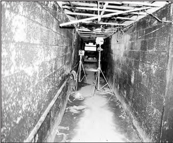
Similarly light fire conditions existed in this hallway on Vandalia Avenue in Brooklyn, where members removed an elderly neighbor prior to conditions suddenly changing and filling the entire 145-foot hall with flame, killing Lieutenant Joseph Cavaliere and FFs Christopher Bopp and James Bohan.
