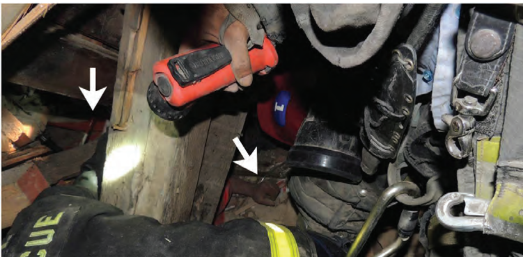
Rescue Operations. Rescuers operating on both sides of the victim meet. On the left center of the picture, you can see one of the small jacks in position to lift (left arrow denotes location). On the right, you can see the victim's left hand, as well as the O2 tube (right arrow denotes location).
