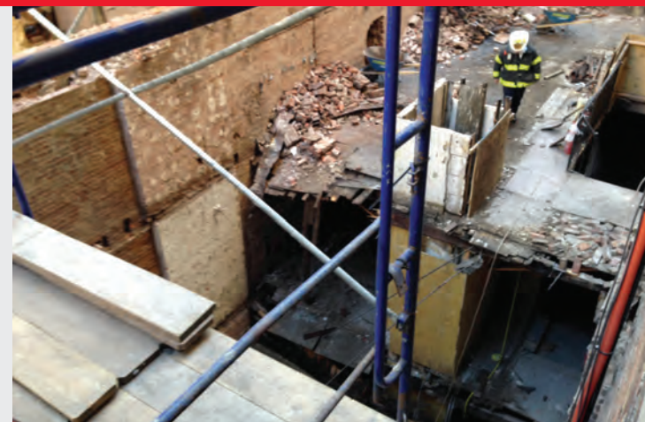
Collapse Factors. Workers stacked bricks on the roof for removal into shafts. Heavy brick piles overloaded the rear of the roof (left). The Safety Chief on the roof was assigned to assist with monitoring the stability of the collapse building (right).
