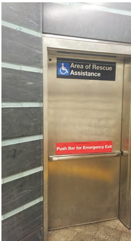
Door for emergency exit.
