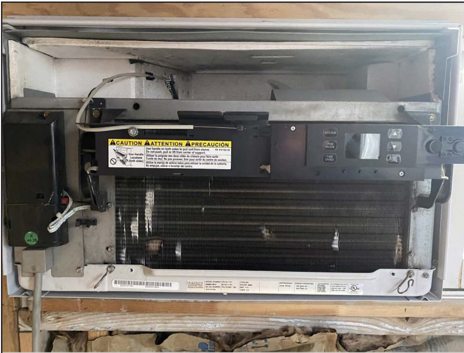
Window-unit evaporator coil. This front coil is where the heat is absorbed into the refrigerant.
