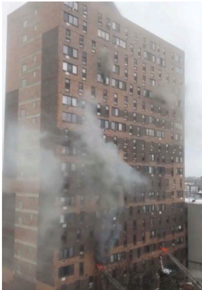
A view of Exposure 1 during the fire. Smoke is emanating from the 15th-floor windows, indicating the severe smoke spread in the fire building because of a chain of open apartment and stairwell doors. (Photo credit: Anjali Singhvi, James Glanz, Weiyei Cai, Evan Grothjan and Mika Gröndahl © 2022 The New York Times Company)
