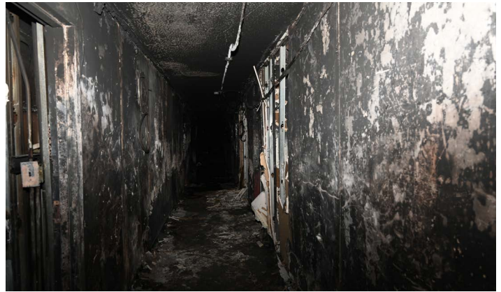
The third-floor public hallway. (Photo credit: Bureau of Fire Investigation)
